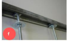
Fix the unistrut into place. There are a range of fixings to accommodate concrete ceiling, girders etc.; if in doubt contact the fixing supplier. Attach the threaded bar to the unistrut using the channel nuts, 38mm washers and M8 nuts. Once this is done the Smoke Screen can be lifted into position and the set screws tightened as above.
