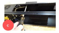
Fit, and ensure tight, 1x M6 set screw with washer in the 2 holes in the back of the Smoke Screen alongside each of the two mounting slots. Access to the fixing holes is through the fluid and heater block compartments.
